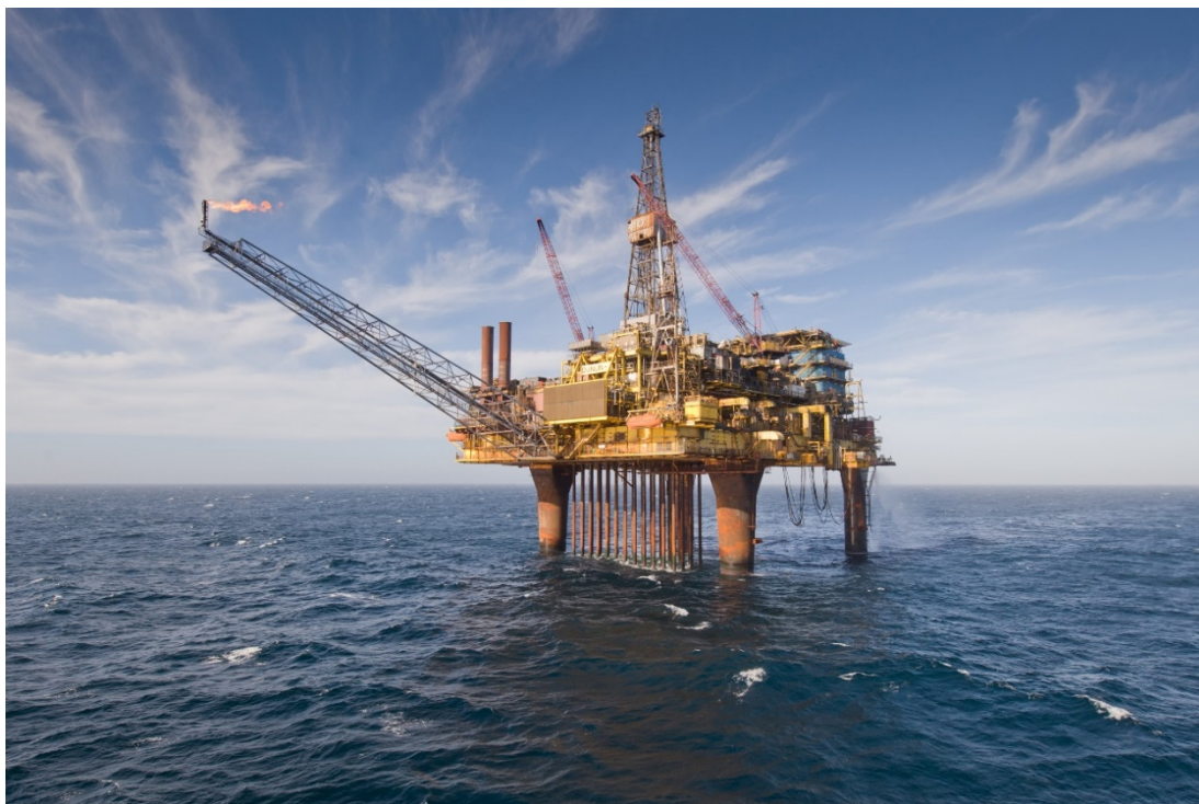
Figure 2-2: Dunlin Alpha Installation (Operational March 2012)
