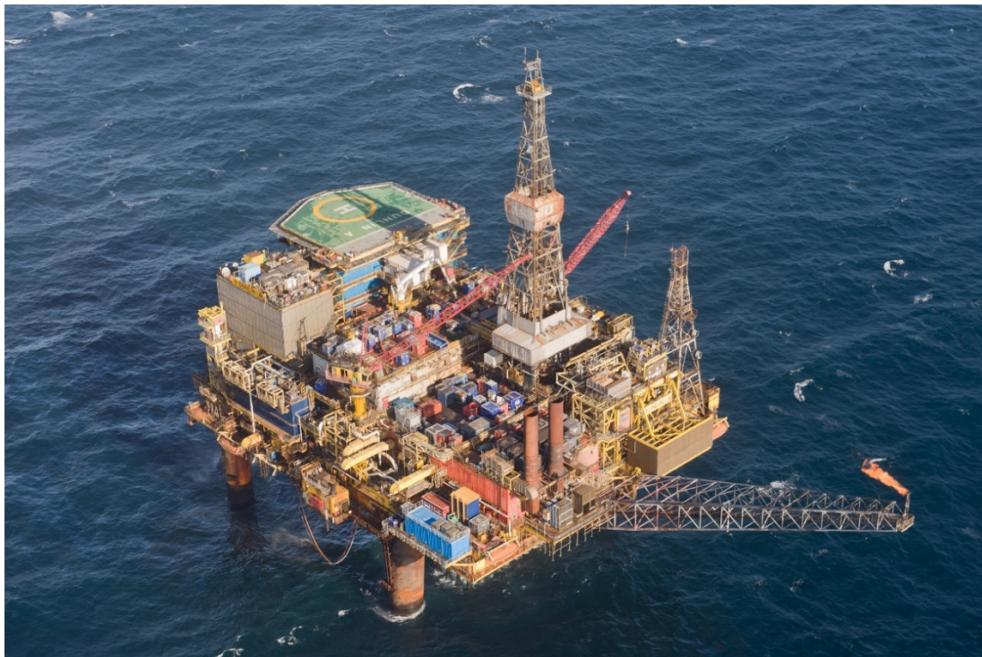
Figure 2-3: Dunlin Alpha Installation (Operational March 2012)
